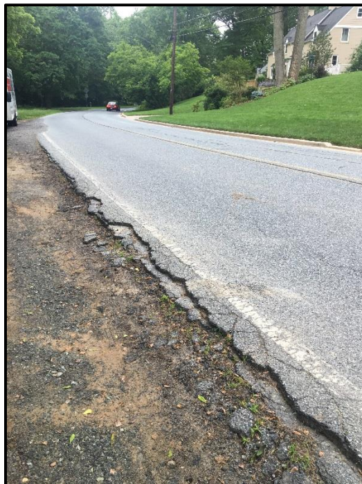
Figure 6. Pavement edge drop off observed along Kensington Parkway
